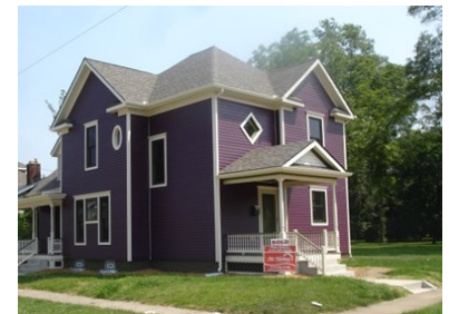
Completed NNN Rehabilitation
