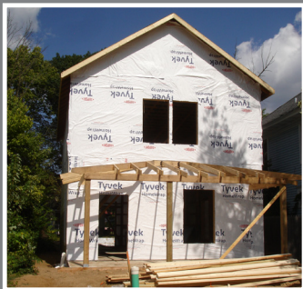
New Home Construction
